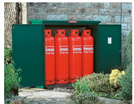
An example of too much gas on the premises. Max 2 x 48kg bottles allowed.
